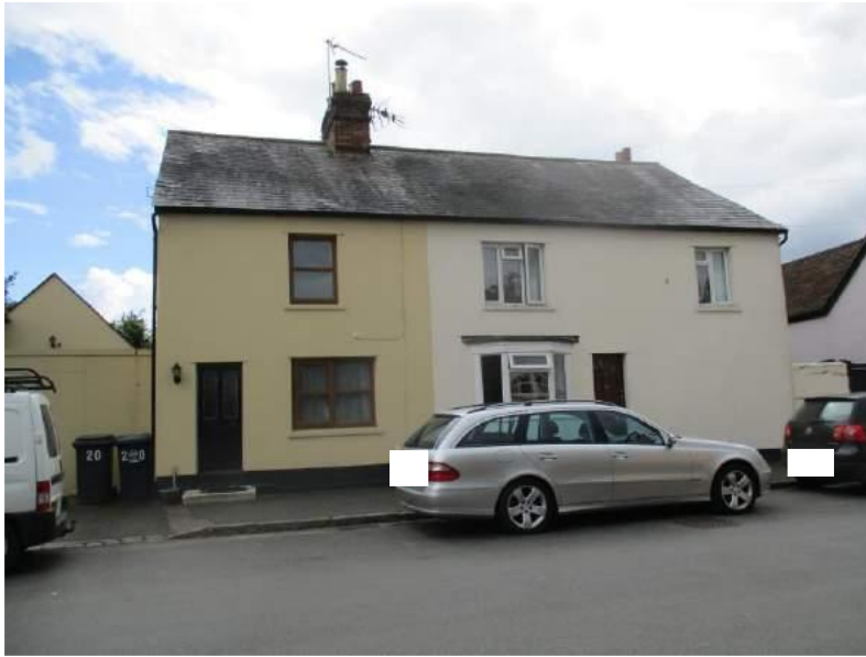
18 and 20 The Street - demonstrating the harm that PVCu windows can have on an historic building.
