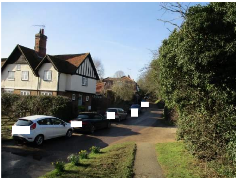
3 Malting Lane and wall with No. 2. Category 1.
